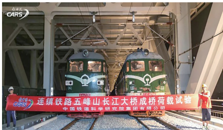
Fig. 10 Wufengshan Yangtze River Bridge completion test
