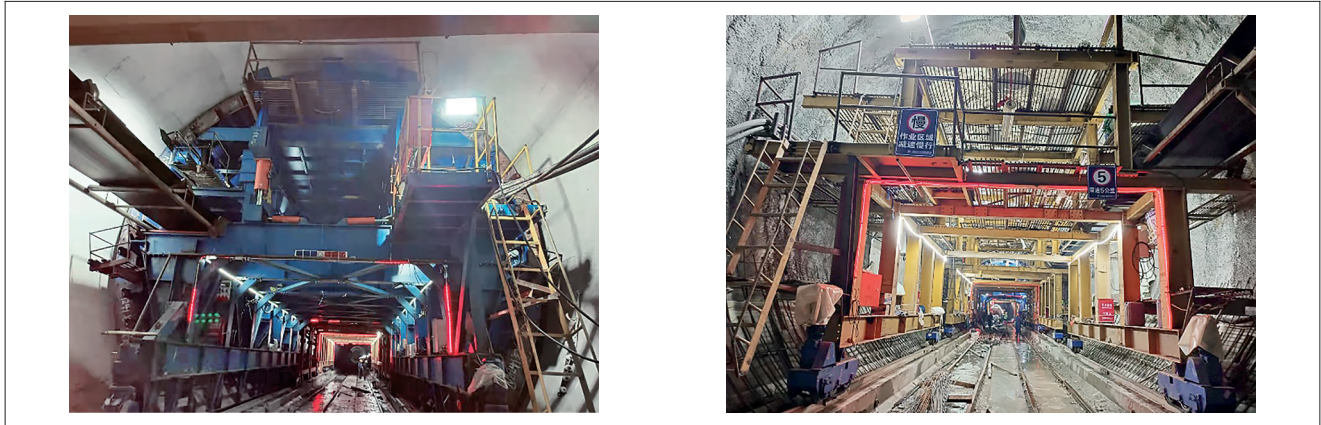
Figure 3 Secondary lining jumbo and rebar bar binding jumbo
