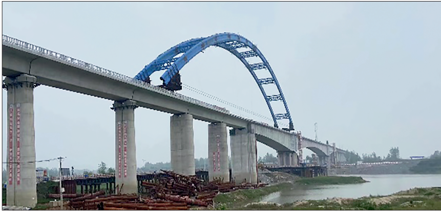
Fig. 5 Actual scene of incremental launching and longitudinal moving
