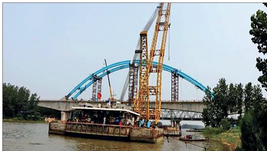
Fig. 2 Site of arch-rib segmental hoisting
